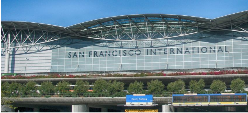
San Francisco Airport – 5 year, $7.3B project
