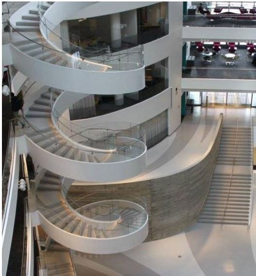
Northeastern University Science Building
